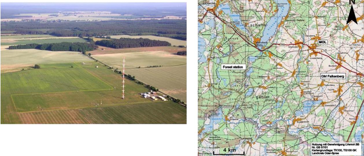
Figure 8 Falkenberg ground site: eddy flux tower (left) and map of the surrounding area (right). The station is identified in the map as “GM Falkenberg”. The tower is 99m height and includes standard meteorological profile measurements (wind speed, temperature, humidity) at levels 10 m, 20 m, 40 m, 60 m, 80 m, and 98 m.
