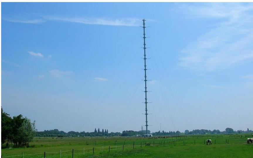
Figure 4 Cabauw site: eddy flux tower and surrounding landscape. The 10, 20, 40, 80, 140, and 200 m heights include observations of air temperature, dew point, relative humidity, specific humidity, wind speed, wind direction, U wind component, and V wind component.
